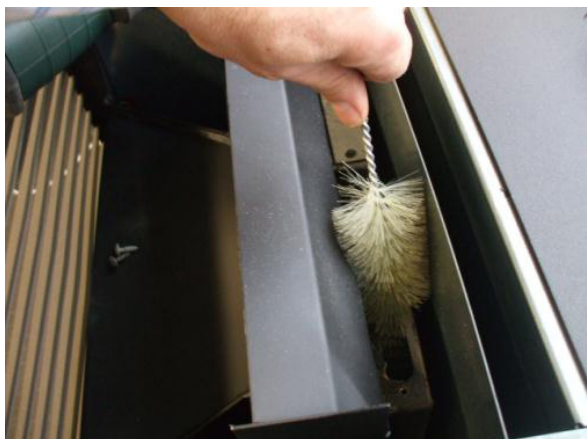
Fig. 40 - Fume passages cleaning
